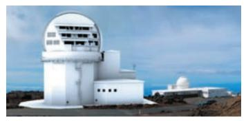
Two computer models illustrate the challenge of maintaining thermal control for ATST. The portrait at left (viewing from the north) depicts ATST at Haleakalā with the vent gates on the carousel open at morning and the telescope pointed east. While it appears se-
